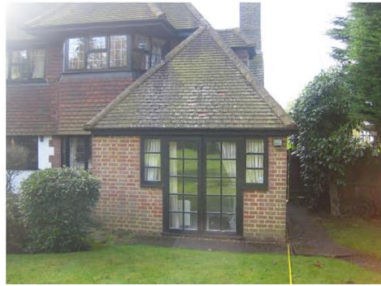
Existing Bricwork and Plain Roof Tile
